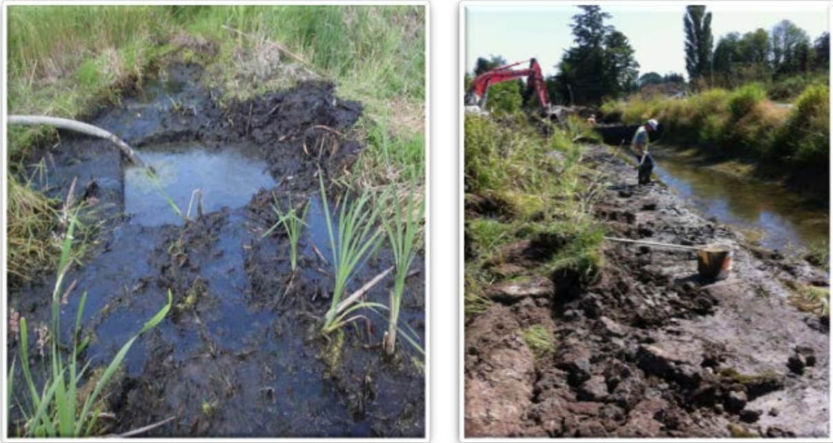
Figure 4. Sump creation and/or pump installation [left; photo credit N. Sands], and dipnetting during dewatering [right; photo credit S. Sloboda]
